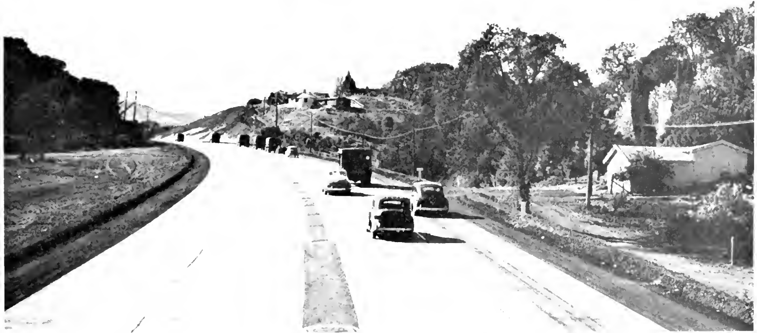
At top, slide section of State Sign Route 24 rebuilt as 4-lane asphalt concrete highway with hydrauger pipe drainage and 3-inch median bars. Below, section over Charles Hill with two 23-foot lanes of Portland cement concrete and 4-foot asphalt concrete dividing strip.
